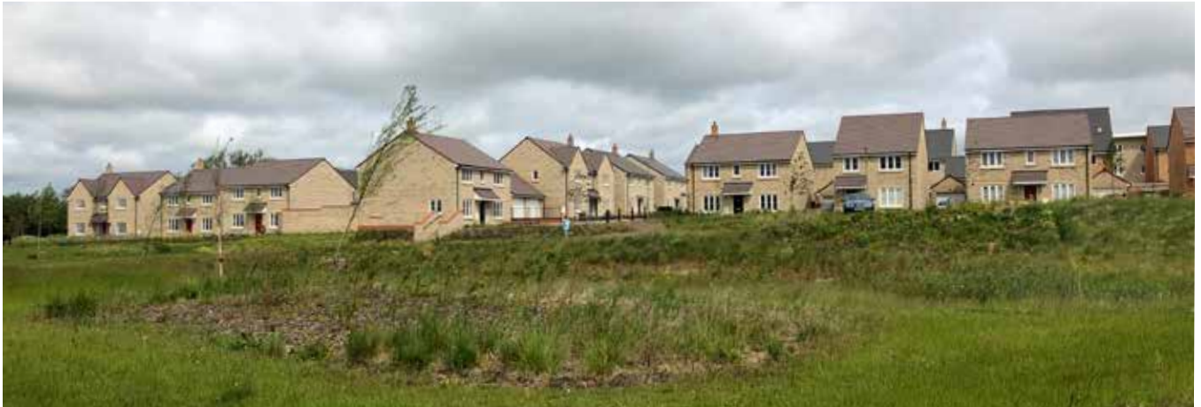
Figure 19: Attenuation feature within Thornbury Green development
