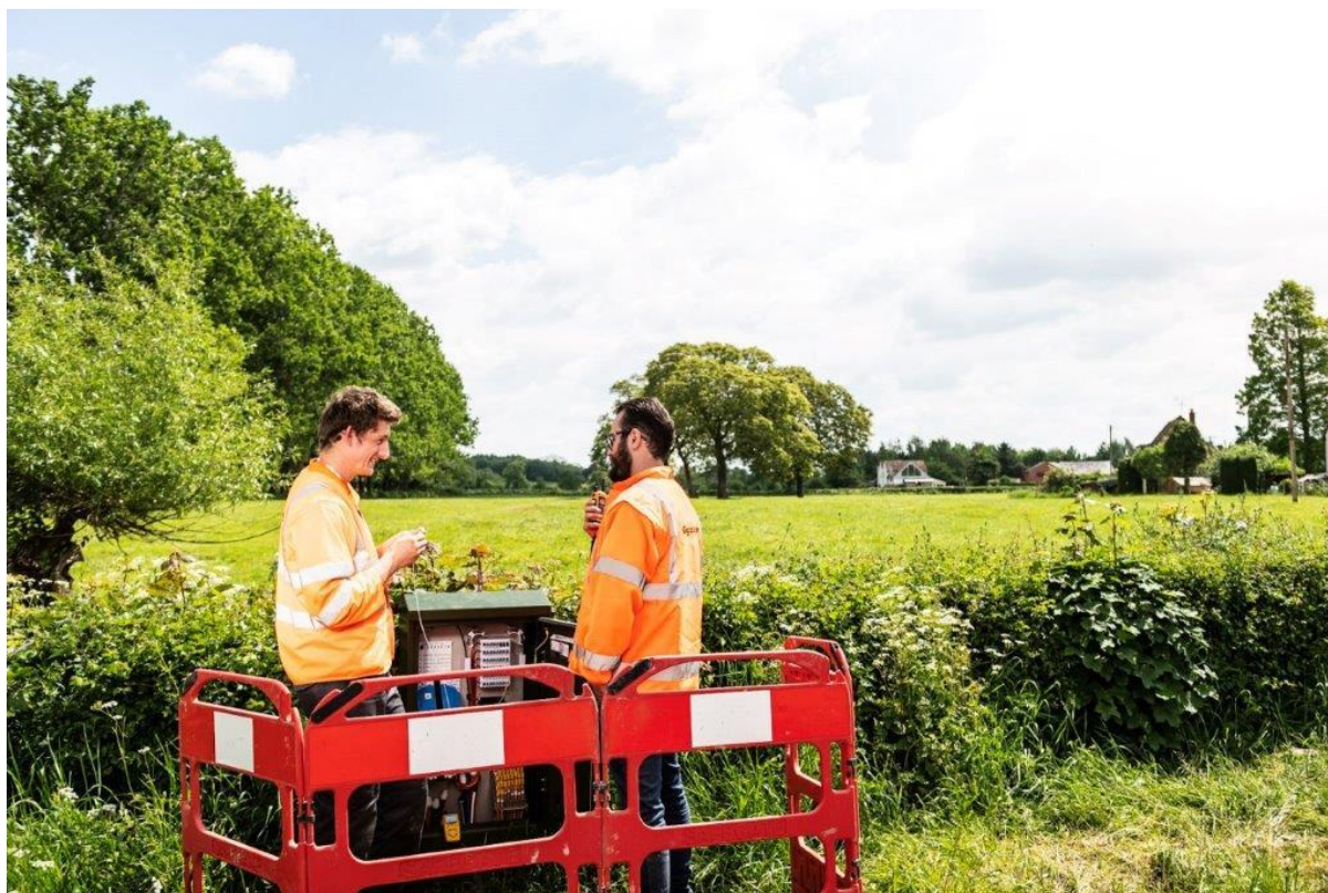
Gigaclear engineers installing a cabinet
