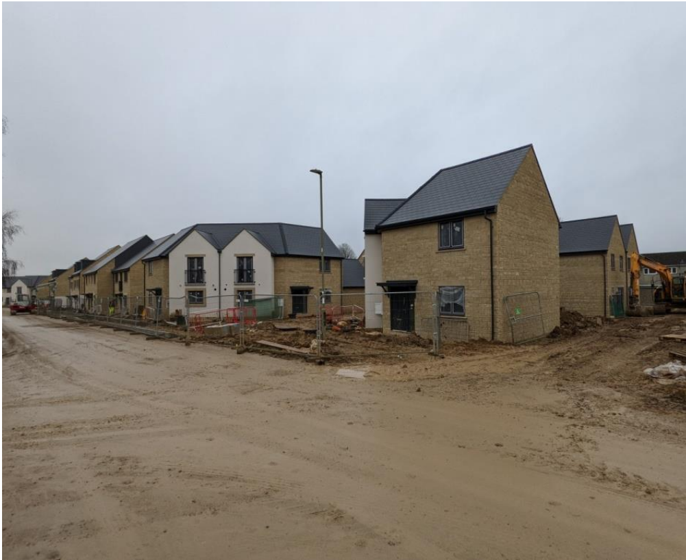
Figure 2: Affordable housing under construction
