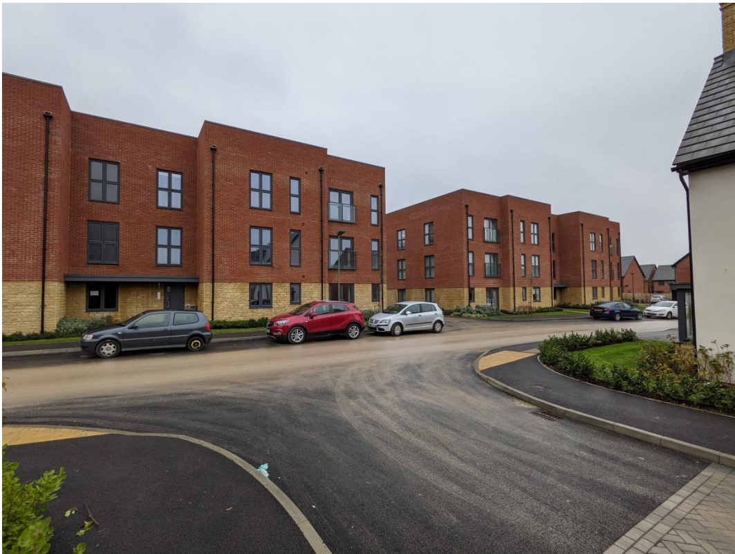
Figure 1: Recently completed affordable housing in West Oxfordshire
