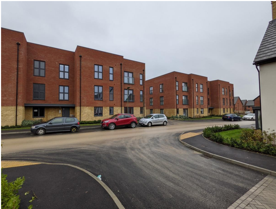
Figure 1: Recently completed affordable housing in West Oxfordshire
