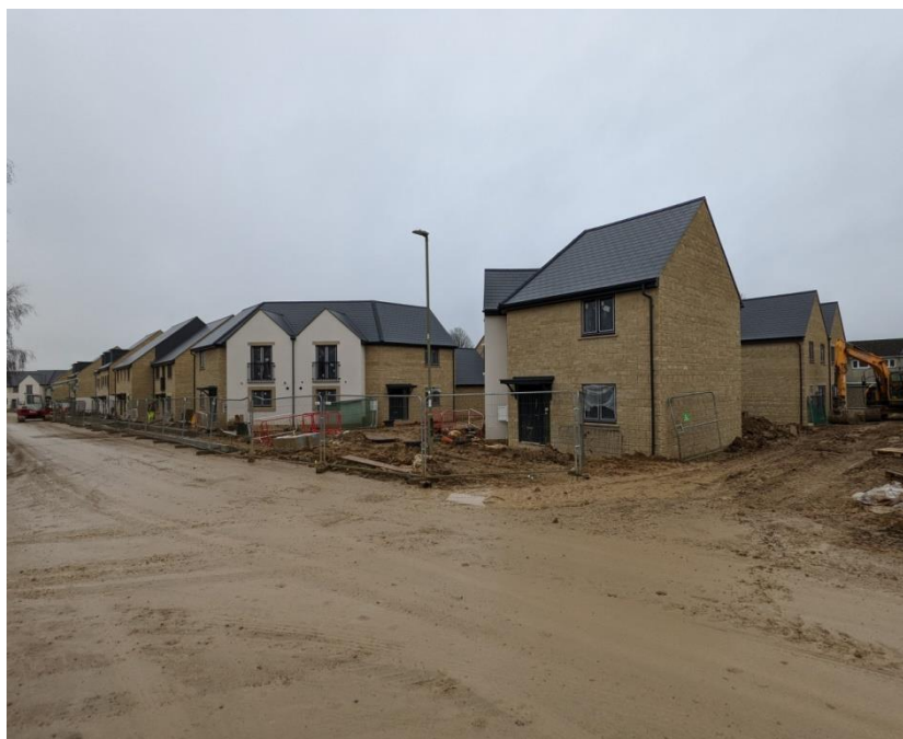
Figure 2: Affordable housing under construction
