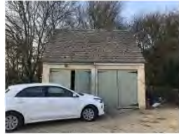
View of Garage Front Elevation
