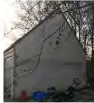
View of Garage Side Elevation (Neighbours)
