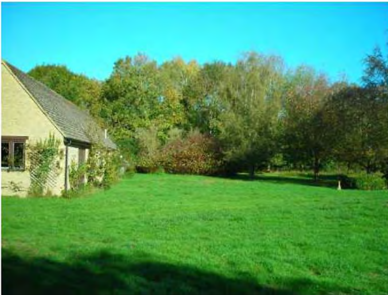
View looking north-east across the site
